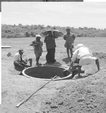
Sinking a Well for potable water
