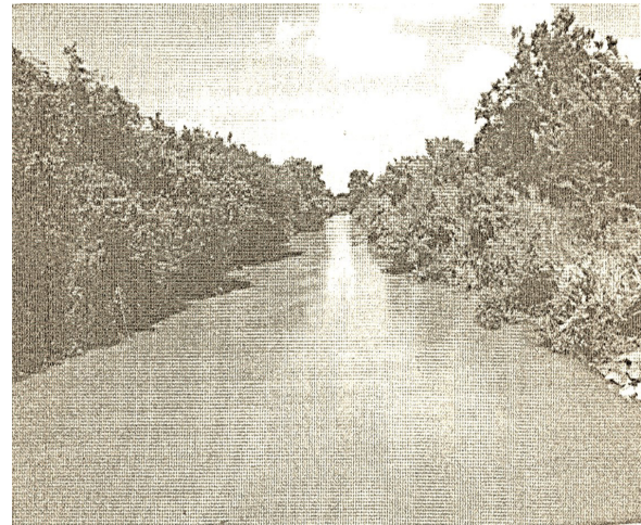
Fig 2 - The Jaya-Ganga (Yoda Ela) that Meanders Through a Natural Thick Forest Ecosystem at an Incredible Gradient of no more than 7 inches per mile in its First 17 Miles. (Reproduced from Awsadahami, 2007)
