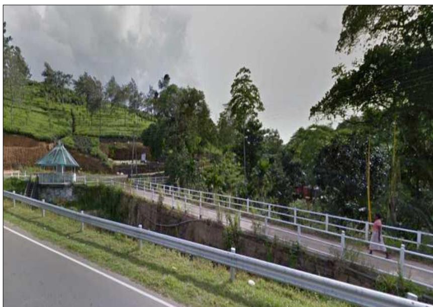
Figure 3. Urubokke Dam and walkway bridge as seen today on the Kotapola-Mulatiana Road.
